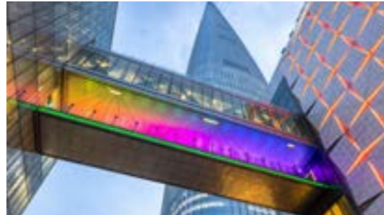
Lotte World Mall Bridge
